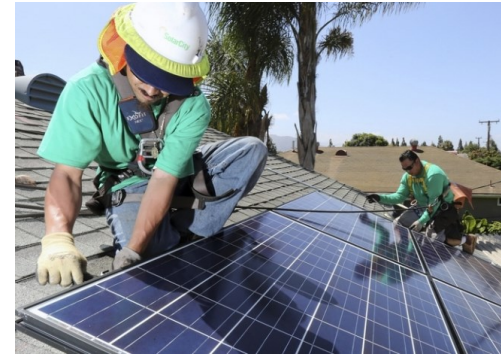
Solar City Employees installing photovoltaic cells on residential homes.
